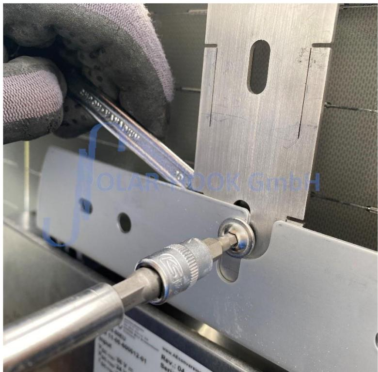
Figure 6 | screw the inverter onto the SOLAR-HOOK mounting bracket
