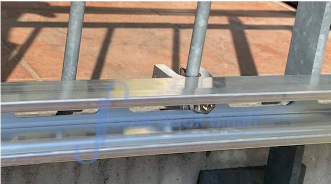
Figure 11/ mounting rail and special clamp from outside
