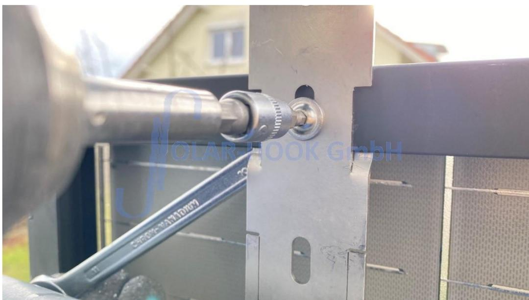
picture 16/tightening the short screws
