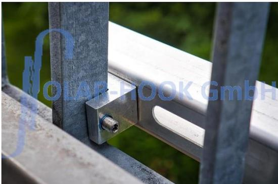
Figure 8b/special clamp on rectangular balcony rod
